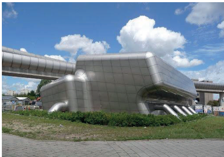
Figura 19. Booster Station , Group A, Amsterdam, 2006
