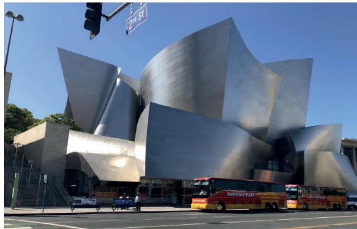
Figura 18. Walt Disney Concert Hall , Frank Gehry, Los Angeles, 2003
